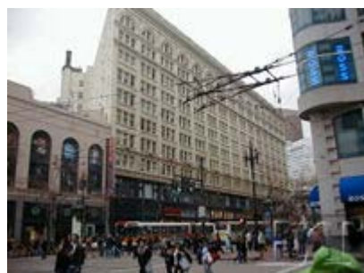
The Phelan Building on Market Street, San Francisco. Dodge's friend James Phelan owned the properties in this area that were purportedly underassessed for property taxes. However, a probe by a grand jury cleared Dr. Dodge of any wrongdoing. © 2002 Jan C. Nielsen. All rights reserved.
